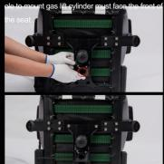
Place the gas lift cylinder with the telescoping cover into the hole at the base of the control mechanism.
